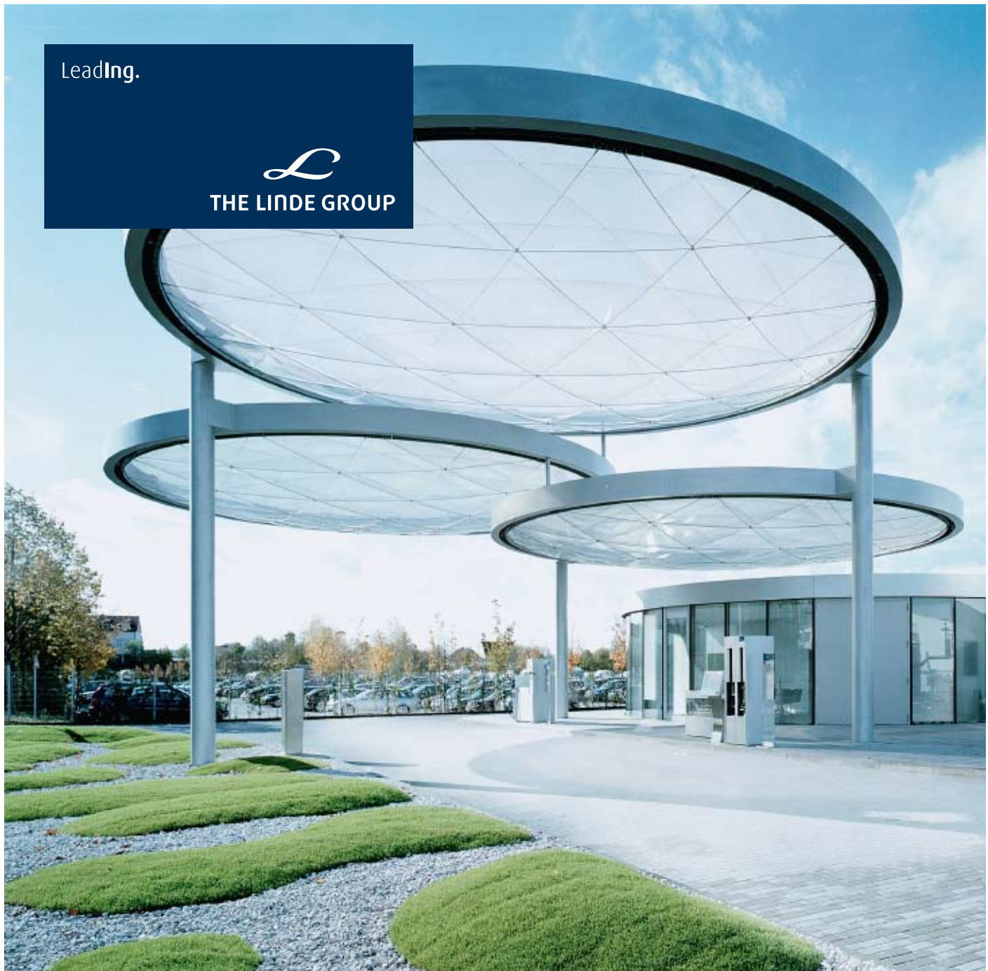
Linde Hydrogen Center in Munich, Germany // Linde Hydrogen Center in München
